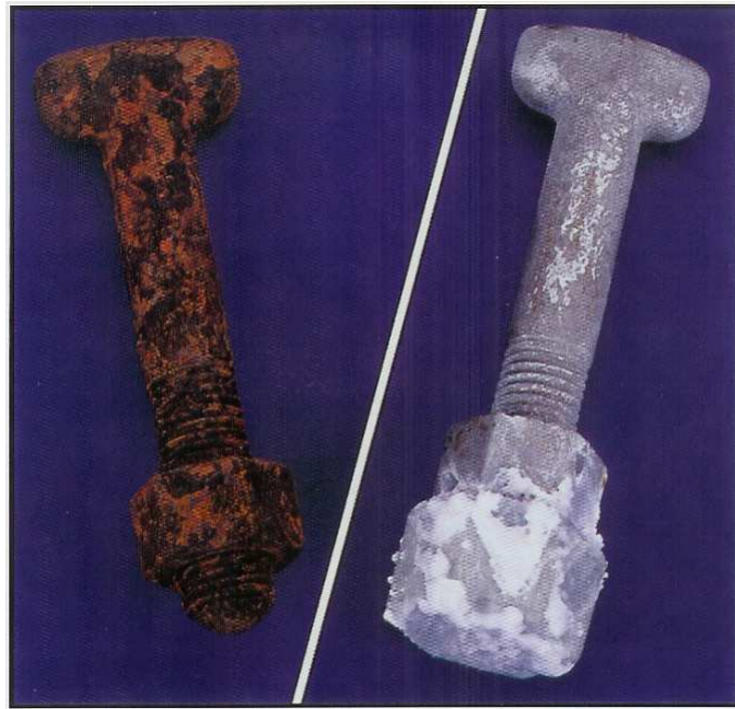
Figure 2.8: After being submerged in concentrated salt water for 5,000 hours, the unprotected iron T-Bolt on the left is totally corroded and unusable.
